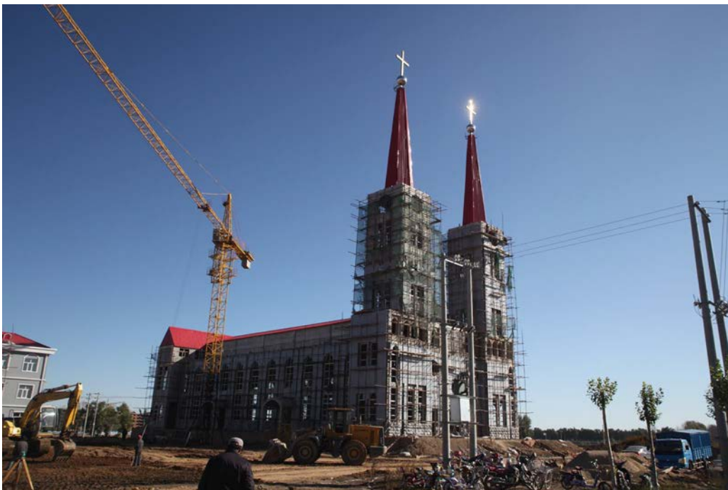
The new church in Zhangbei under construction. Photo: Zhangbei parish.
